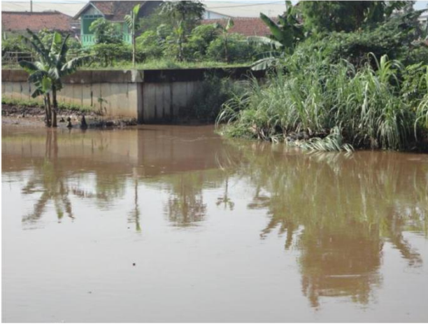
Figure 2.11: Flood wall along Citarum river near Cieunteung (March 2016)
