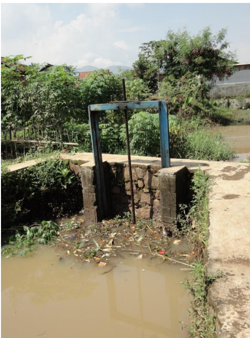
Figure 2.13: Gate in drain at Cieunteung (March 2016)
